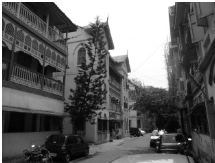
Lal Chimney prior to restoration.
