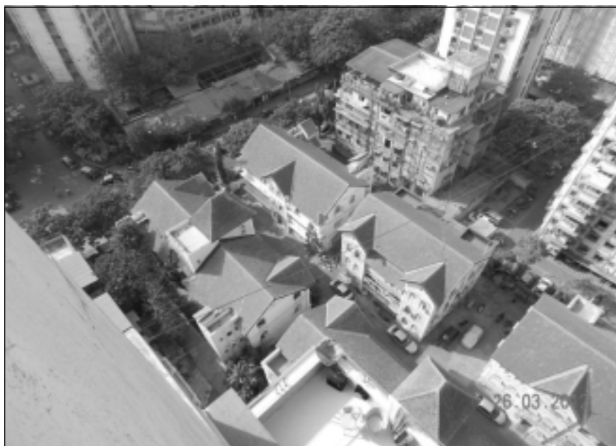
Lal Chimney ariel view post restoration.
